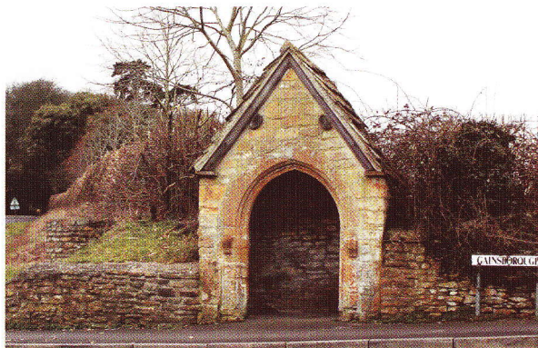
The pump house and well
